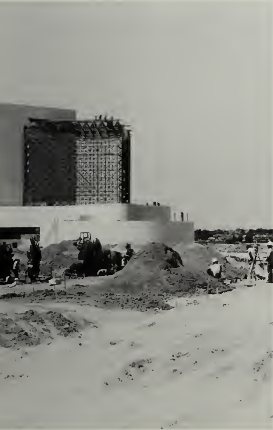
Finishing construction of the Kennedy Library, 1979. Courtesy of the Boston Globe.
